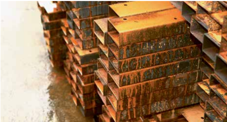
Fig. 4: Corrosion of steel components.
