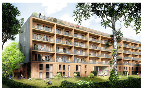
Engineered wood construction (sample)
