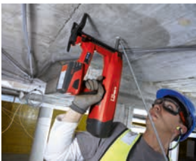
Threaded rod attachments to concrete
