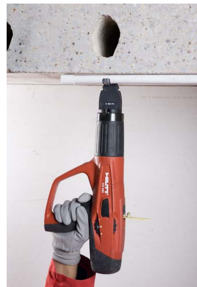
DX 460 being used for fixing electrical conduit.
