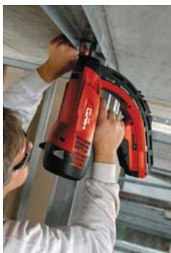
Securing head track with gas tool
