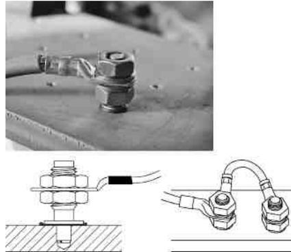
Figure 80. Grounding point provided by a blunt tip stud
