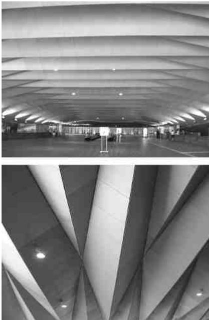
**Figure 82.** The nailed folded-sheet structure of the ship terminal at Yokohama
