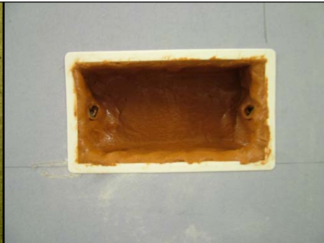
Photograph 4. Hilti Putty Pad fitted into wall box
