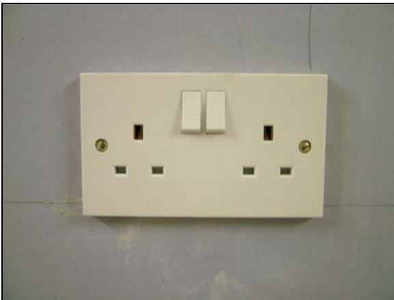
Photograph 5. Socket fitted to wall box
